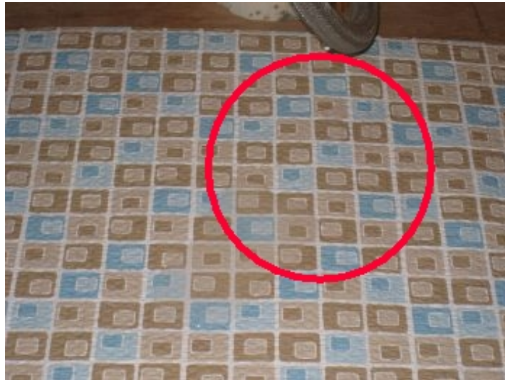
Water leak under kitchen sink
