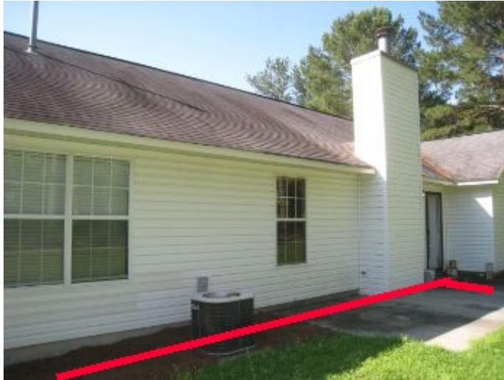
Rear roof drainage area
