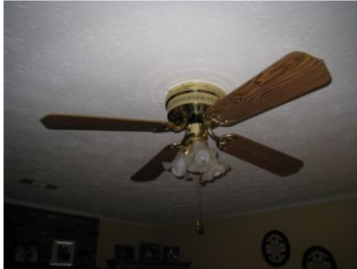
Noisy ceiling fan in family room
