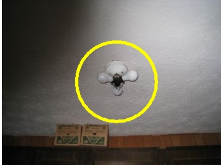
Bare bulbs in utility room
