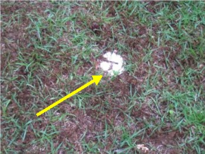
Waste pipe clean-out in front yard
