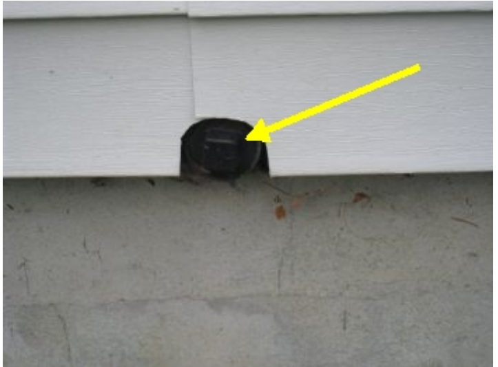
Waste pipe clean-out at rear of house
